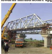
Central Railway, continuing its strides towards infrastructure upgradation, carried out launching of 30.5-meter span open web girder weighing 100 MT of Rail Fly Over on Bhadli-Jalgaon 4th line (part of Jalgaon-Bhusaval 24km - 4th line project) on 12.1.2022. The main girder was launched by end-
